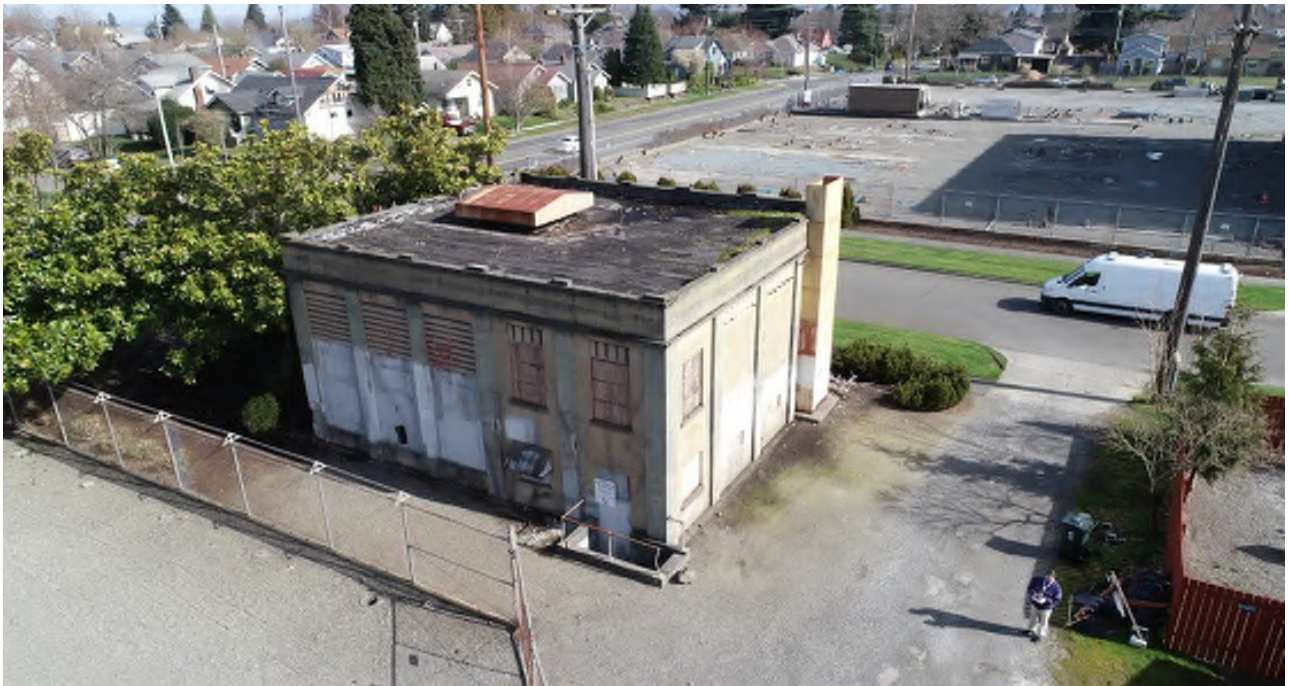
Adams Substation West and South elevations.
