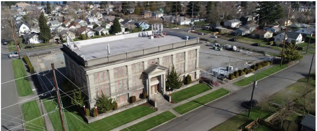
Present-day photo of the Cushman substation building and site
