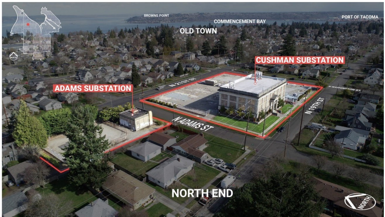
Figure 3—Bird’s Eye Aerial View of Substation Sites
